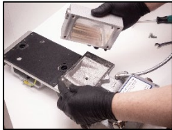
5. Replace the valve box gasket.
