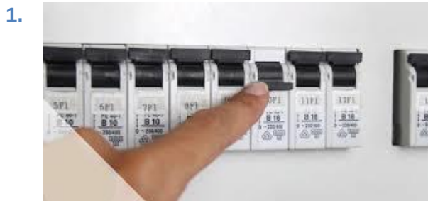
Figure 151: Switch off the power supply
