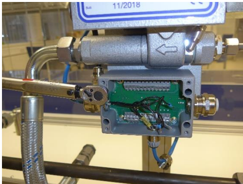
Figure 119: Install the terminal box
