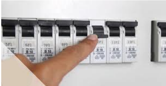
Figure 115: Switch off the power supply
