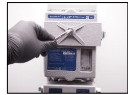
12. Disconnect the u-tube manometer and install the plug for inspection cover.
