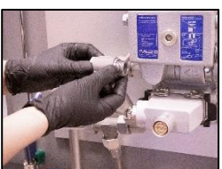
2. Remove the pipe from oil mist detector.
