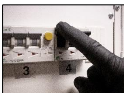
1. Turn off the power to the oil mist detector.
