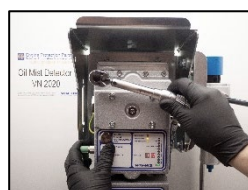
3. Replace the measuring head. Tighten the captive screws crosswise with torque of 4.5Nm.
