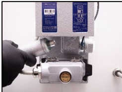
1. Disconnect the ejector output.
