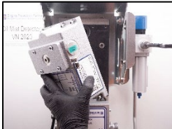
1. Disconnect the measuring head from the base plate.
