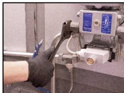
1. Loosen the main pipe connection.
