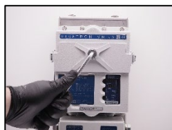
18. Change the screw plug seal \frac{1}{4} " for inspection cover (Part nr.: 10082).
