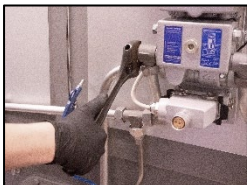
1. Loosen the main pipe connection.
