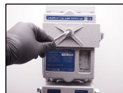
19. change the screw plug seal 1/4" for inspection cover (Part nr.: 10082)
