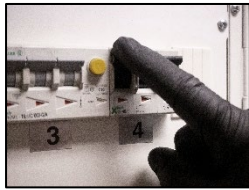
1. Turn off the power to the oil mist detector
