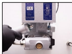
1. Disconnect the ejector output
