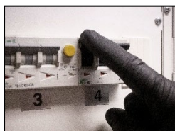
1. Turn of the power to the oil mist detector
