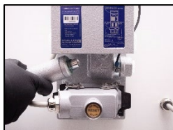
1. Disconnect the ejector output
