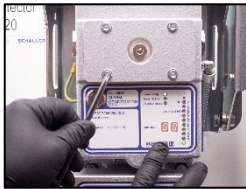
1. Remove the plug in the inspection cover.
