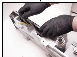
9. Install the pipe connection box.
