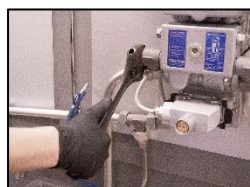
1. Loosen the main pipe connection.
