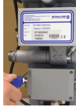
Figure 49: Install the cover on terminal box
