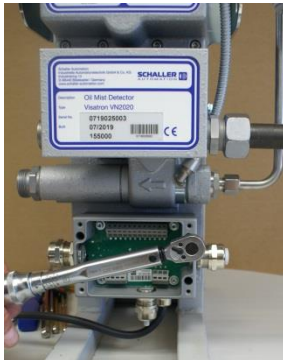
Figure 136: mounting of terminal box
