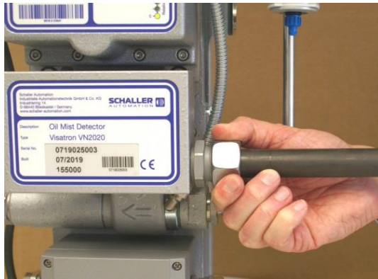
Figure 89: mounting of header pipe
