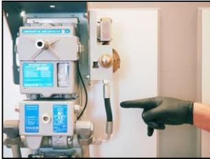
1 Start with disconnecting the flexible main tube from the base plate to the regulator...
