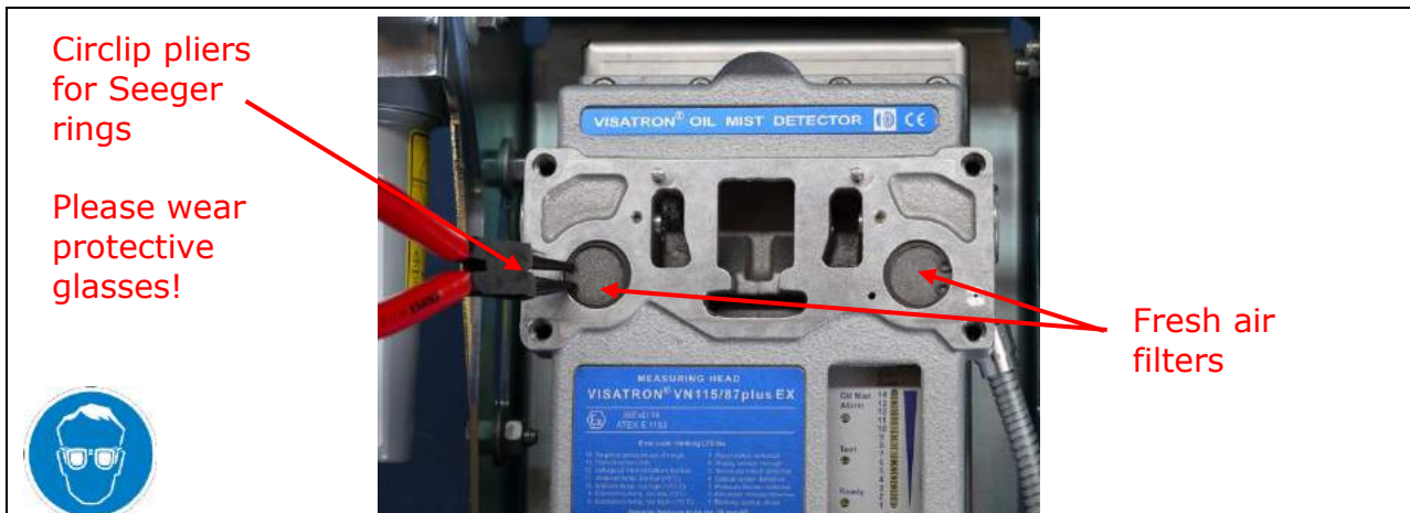
Figure 36: Exchange of the air filters
