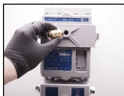
7. Install the quick connection.
