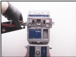
2. Replace the sintered bronze air filter/fresh air filter.
