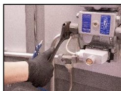
1. Loosen the main pipe connection.
