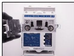
13. Open the inspection cover.
