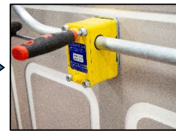
4. Loosen the screws on the siphon block...
