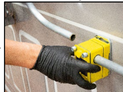
6. Disconnect the pipes from the siphon block.
