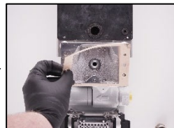
6. Check the valve box seal.
