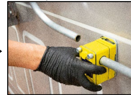
12. Re-connect the pipes to the siphon block.
