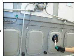
3. Repeat the process for all the sampling funnels to ensure the pipe is not blocked. Use the same tube as long as it is producing smoke.
