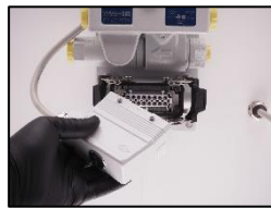
2. Disconnect the RESET task connector.
