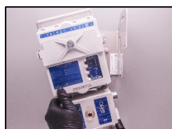
2. Disconnect the used oil mist detector.
