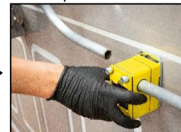
12. Re-connect the pipes to the siphon block.
