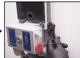
8. Unscrew the vibration plate...
