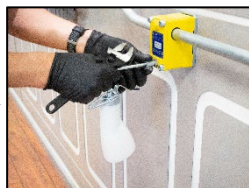
14. Insert pump into the siphon block.
