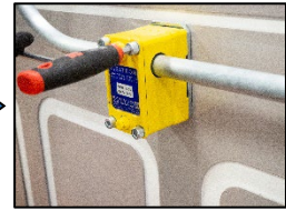
4. Loosen the screws on the siphon block...
