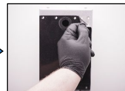
12. Change the measuring head seal.
