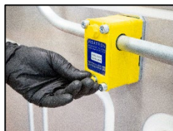
13. Unscrew the bottom screw on the siphon block.
