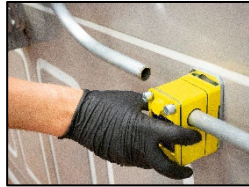
6. Disconnect the pipes from the siphon block.
