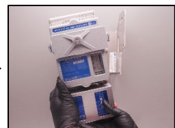
4. Install new exchange unit and main connection socket.
