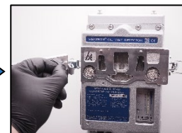
16. Change the seal for inspection cover.
