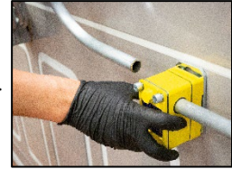
12. Re-connect the pipes to the siphon block.
