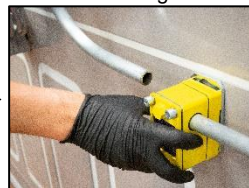
6. Disconnect the pipes from the siphon block.
