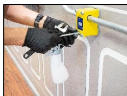
14. Insert pump into the siphon block.
