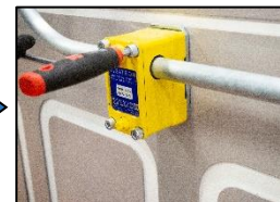
4. Loosen the screws on the siphon block...
