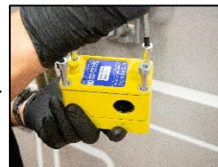
7. Unscrew the screws completely
