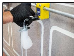
15. Tighten the screw on the pump.
