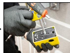
8. Take of the cover of the siphon block.
