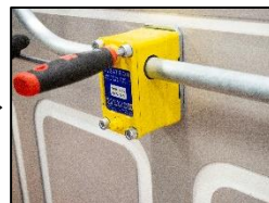
4. Loosen the screws on the siphon block...
