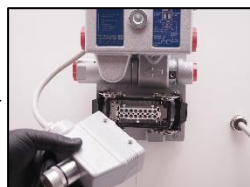
2. Disconnect the RESET task connector.
