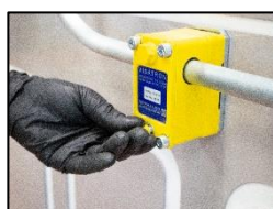
13. Unscrew the bottom screw on the siphon block.
