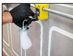
15. Tighten the screw on the pump.
