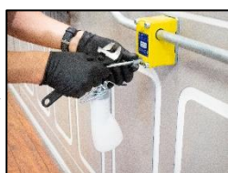
14. Insert pump into the siphon block.
