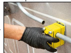
12. Re-connect the pipes to the siphon block.
