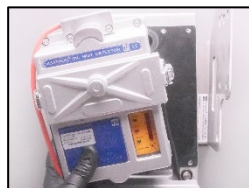
14. Replace the measuring head.
