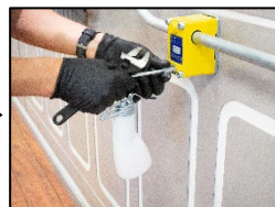
14. Insert pump into the siphon block.
