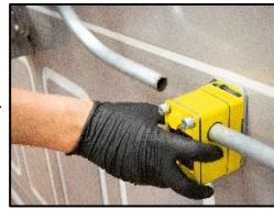
6. Disconnect the pipes from the siphon block.
