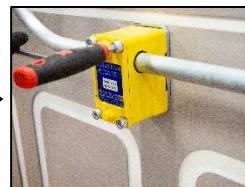
4. Loosen the screws on the siphon block...
