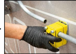
12. Re-connect the pipes to the siphon block.
