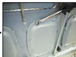
4. When all sampling funnels have been tested, close the crank case covers and your system is ready for use.
