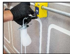
15. Tighten the screw on the pump.
