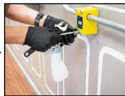
14. Insert pump into the siphon block.
