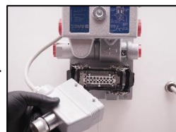
2. Disconnect the RESET task connector.
