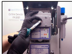
5. Pump smoke until the oil mist alarm is realised.
