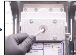
12. Disconnect the u-tube manometer and install the plug for inspection cover.
