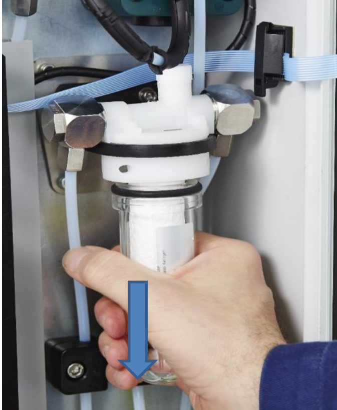
Figure 53 Removing the filter bowl
